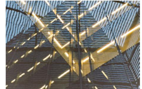
Toughened glass may show visual distortions which are accentuated by reflections in sealed units. This is a natural phenomenon and not a fault.
